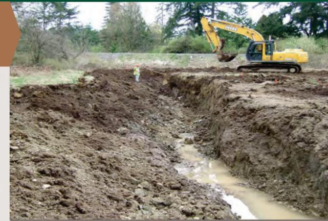
Excavating the new stream bed before the stream was transferred.
