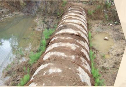
*At this location, Wray Creek was once enclosed in an old wooden culvert dating back to approximately 1968. The pipe was failing and it was decided to “daylight” the creek by removing it from the pipe and restoring habitat.*
