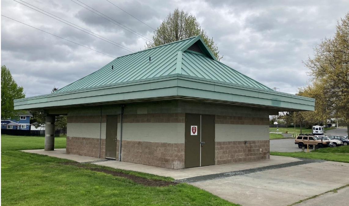
Beckwith Park: South and East Walls
