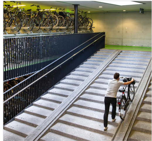
Figure 38: Stairs that include a ramp and small channel for bicycle wheels (3.4.2. o).
