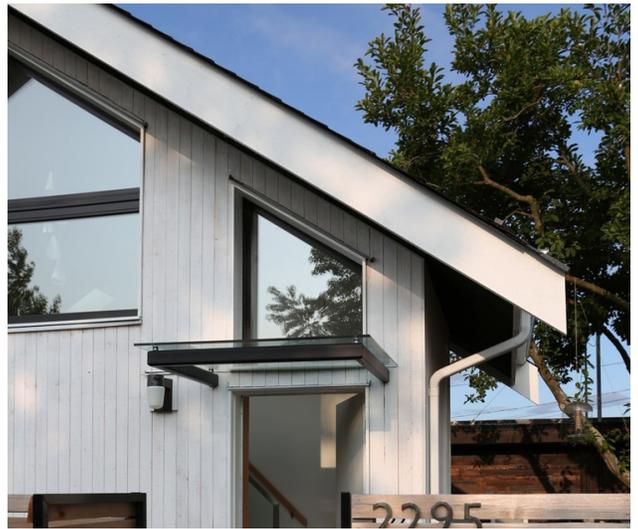
Figure 12: A covered entry to a garden suite provides weather protection.
