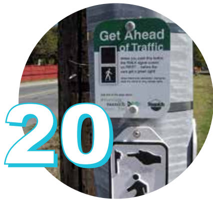
Traffic signals upgraded to give more pedestrian priority through Leading Pedestrian Intervals
