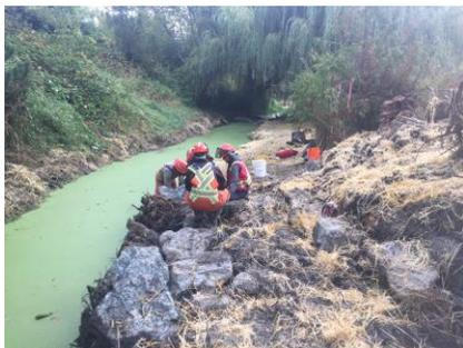
Working with the Public Works Creeks & Waterways crew, a large section of Swan Creek (off Columbine) has had significant work done to increase flow and improve the habitat for fish spawning. Several yards of spawning gravel was placed in the creek bed plus a small section of large boulders and stumps were added for bank stability and fish habitat.
