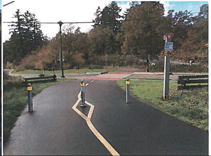
Why are outer bollards placed within path. Silver bollards are not very visible compared to white bollards.
