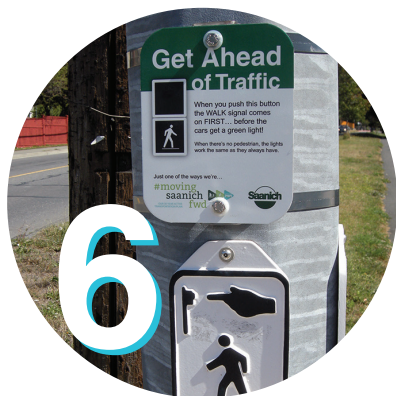
Traffic signals upgraded to give more pedestrian priority through leading pedestrian intervals
