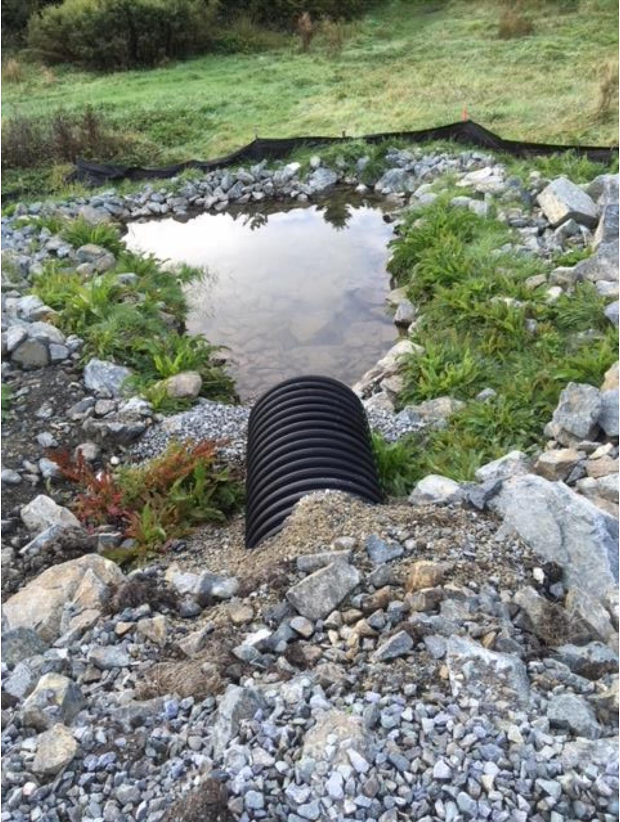
Rock pit to manage storm water flow from other side of highway, September 12, 2018.
