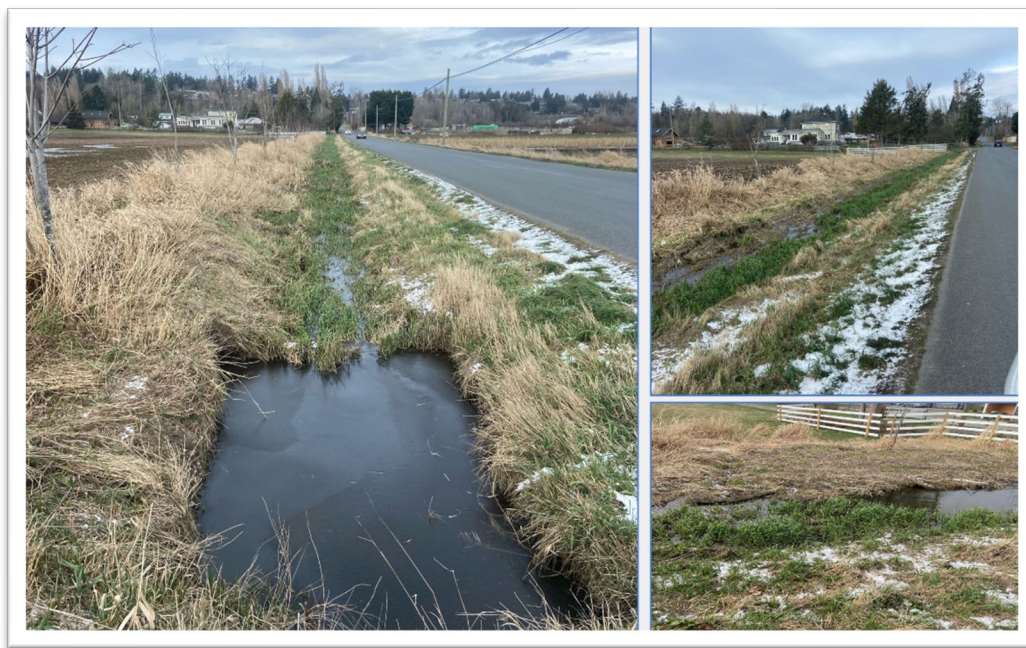
Drainage on Martindale Flats
