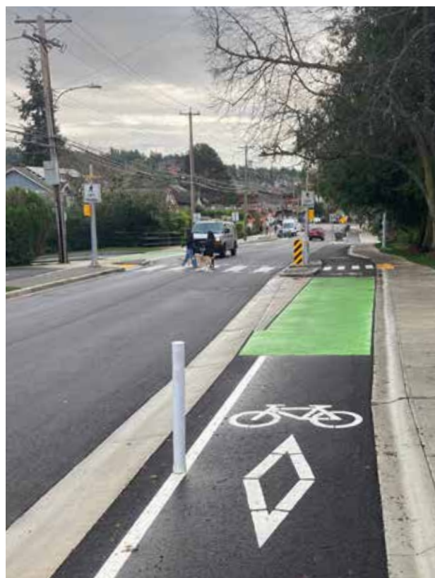
Newly completed crosswalks, sidewalks, and, bike lanes on Sinclair
