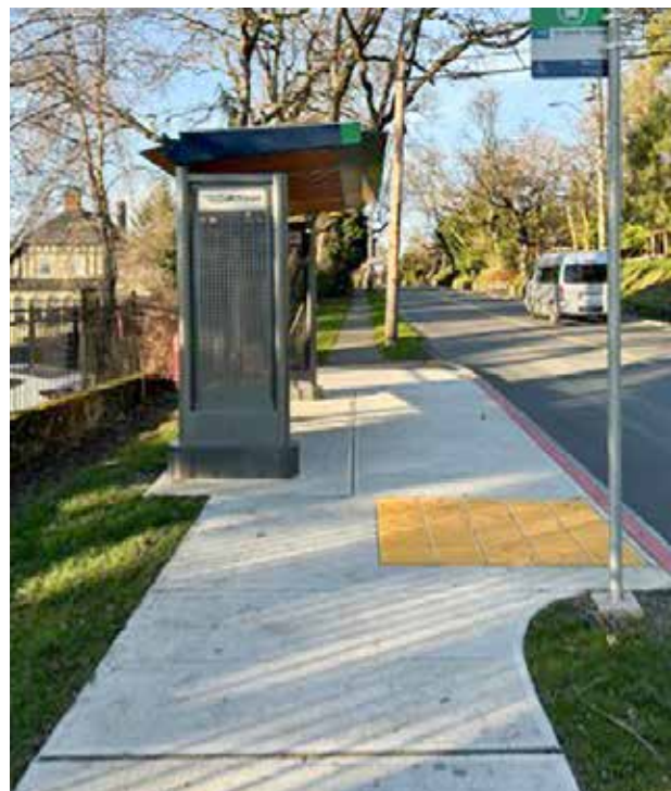
Bus stop improvements at Richmond SB McRae
