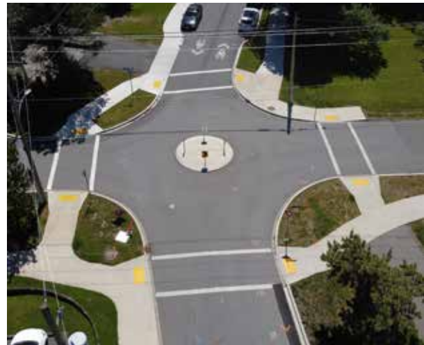
Completed Seaton-Regina sidewalk project
