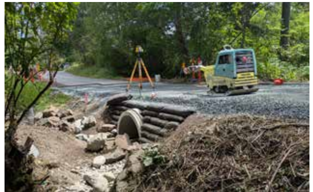
Preparing to pave Charlton Road
