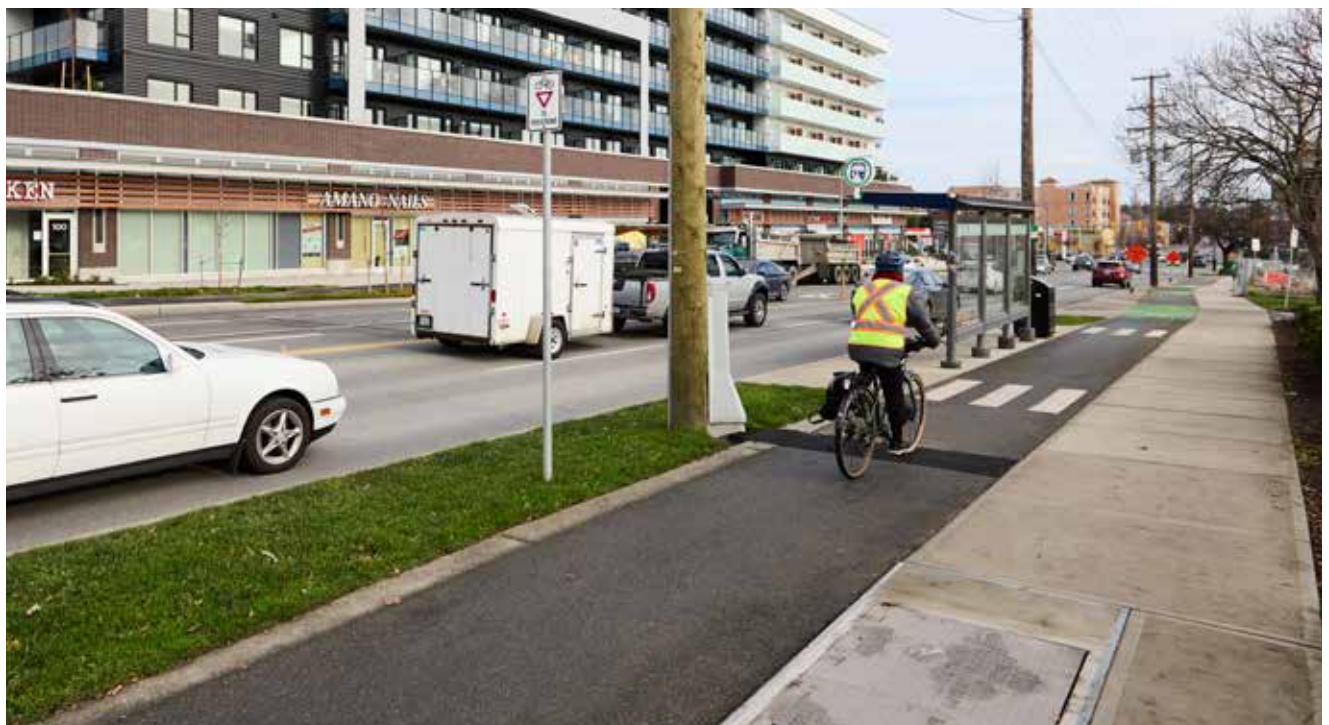
McKenzie Avenue upgrades include a protected bike lane
