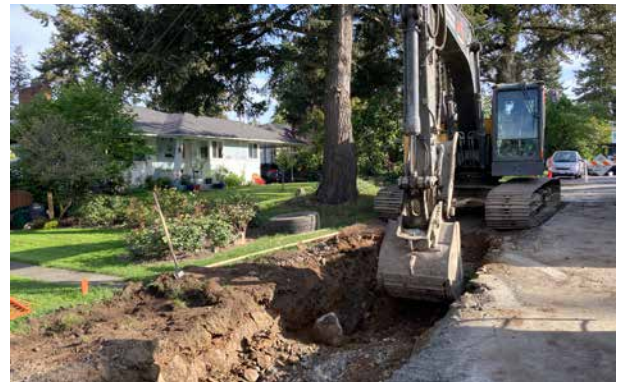
Excavating on Adelaide Avenue - preparing for bedrock removal during storm drainage main installation
