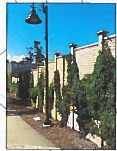
CONCRETE FENCE 2.5m HIGH
