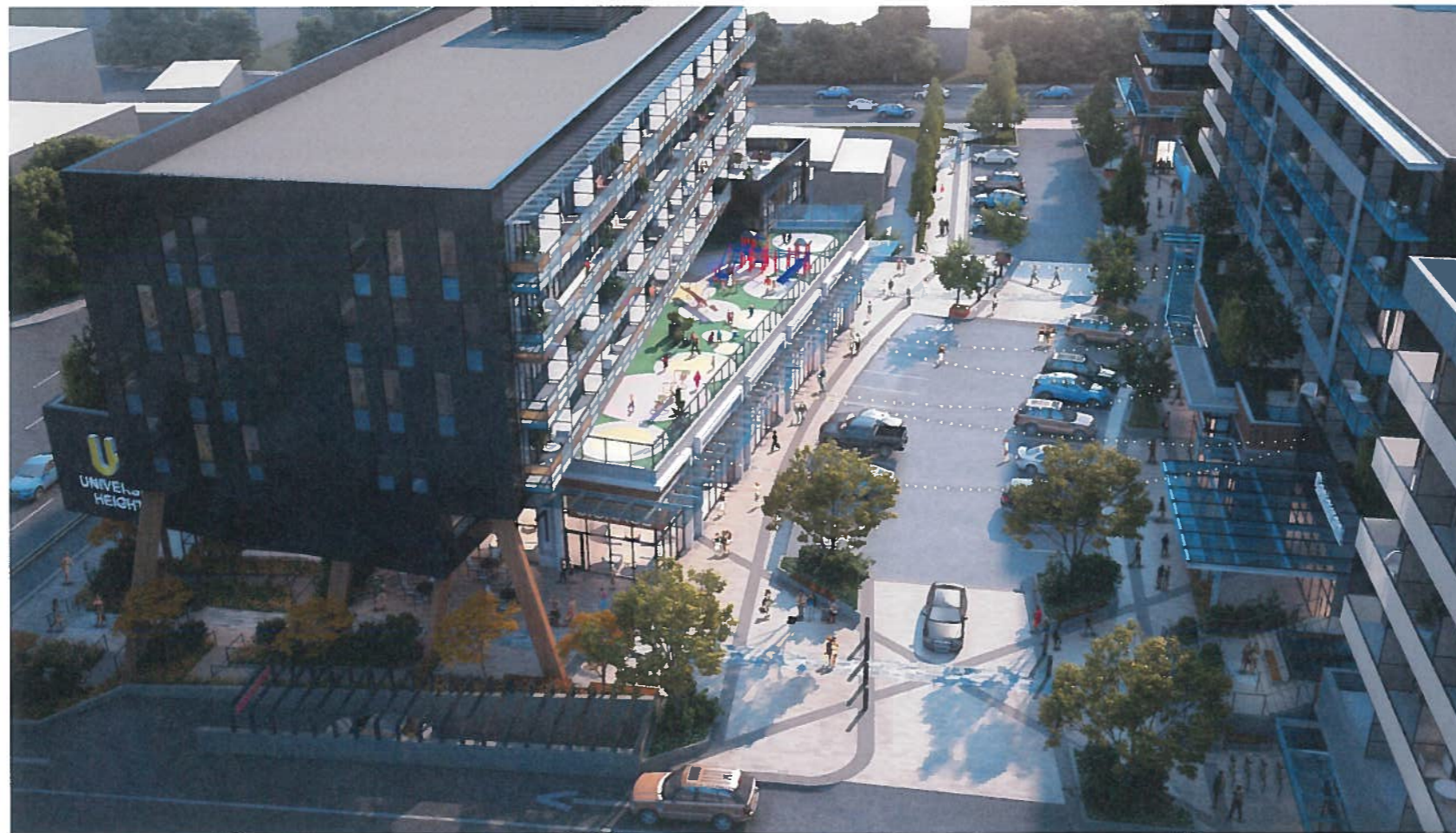
2 AERIAL VIEW OF DAYCARE ROOF AND HIGH STREET ADDN HTS
