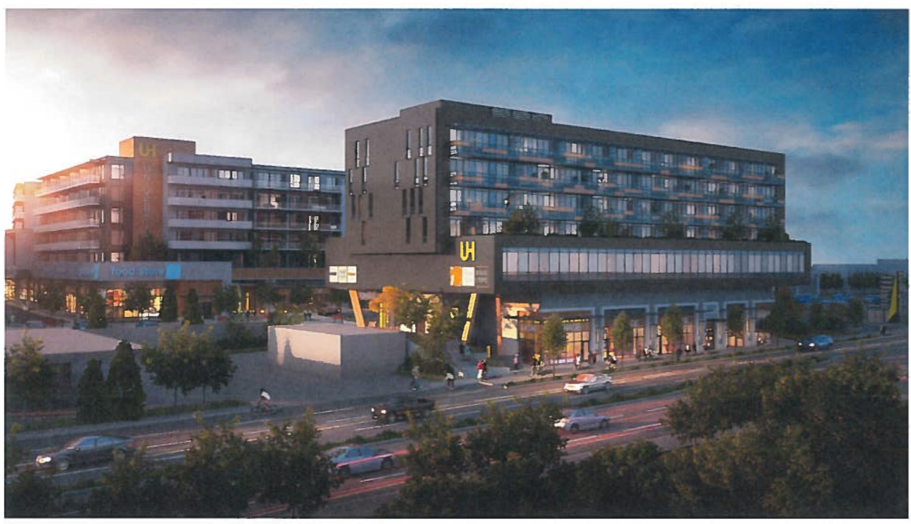
1 VIEW OF SHELBOURNE FRONTAGE LOOKING NORTHWEST
