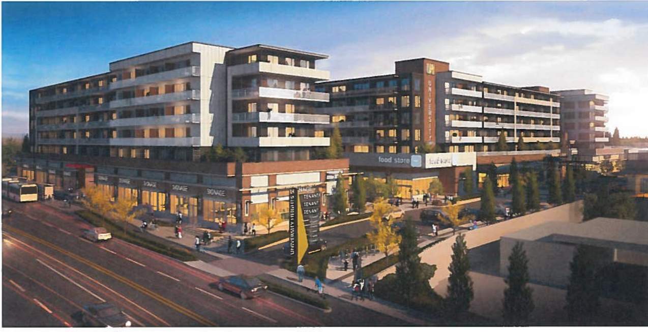
2 VIEW OF MCKENZIE FRONTAGE LOOKING NORTHWEST ADD N/A
