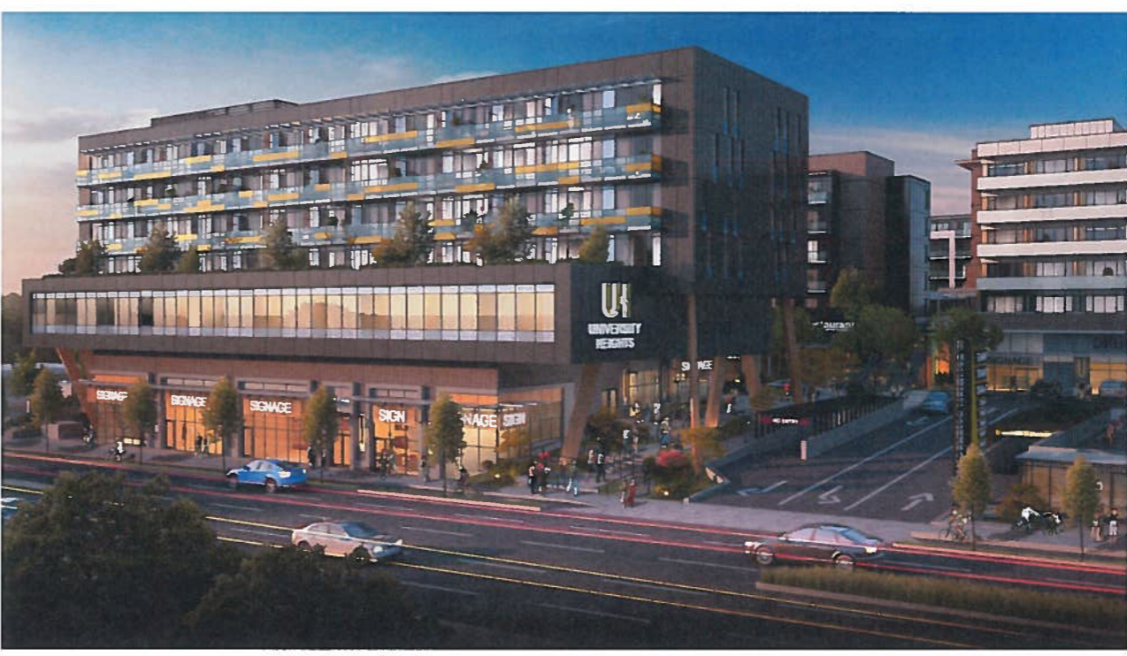
2 VIEW OF SHELBOURNE STAIR LOOKING SOUTHWEST
