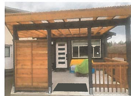
Existing Building as shown
