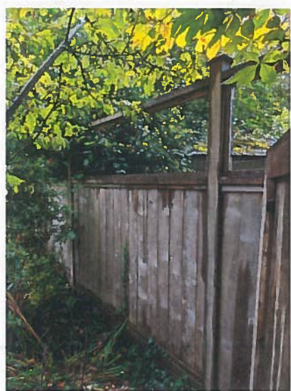
VIEW OF EXISTING FENCE ON SOUTH PROPERTY LINE, AT GARDEN SUITE SITE. FENCE PANELS ARE 1.2m HIGH, WITH AN ADDITIONAL 0.6m METAL MESH, TOTAL HEIGHT: 1.8m (6'-0")
