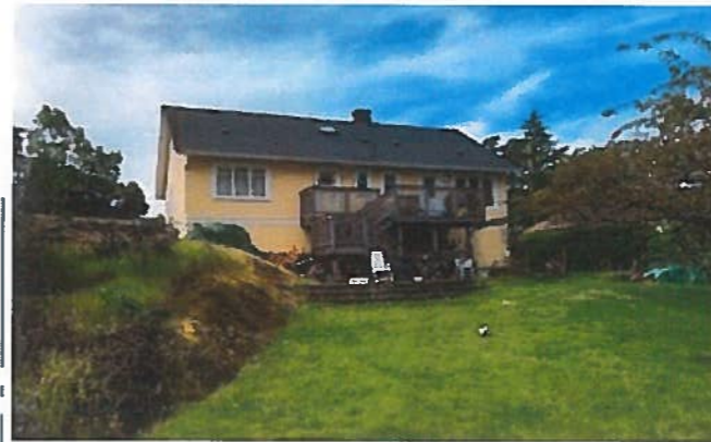
North Side - Existing Residence
