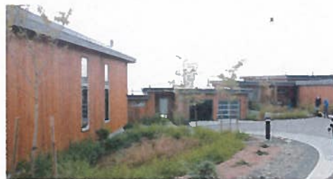
Ophir Street Streetscape: Road runoff from Ophir Street cul-de-sac to be directed to rain gardens in landscape bays, planted with Tulip trees and mixed shrub and perennial planting.
