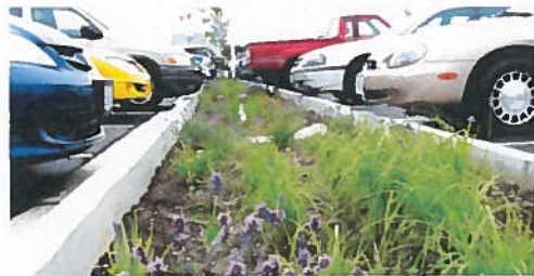
Parking Lot: Concrete unit pavers sloped to run off into swales and rain gardens. Wheel stops placed 1m back from end of parking stall to create more planting space. Plantings include Douglas fir and Katsura trees.
