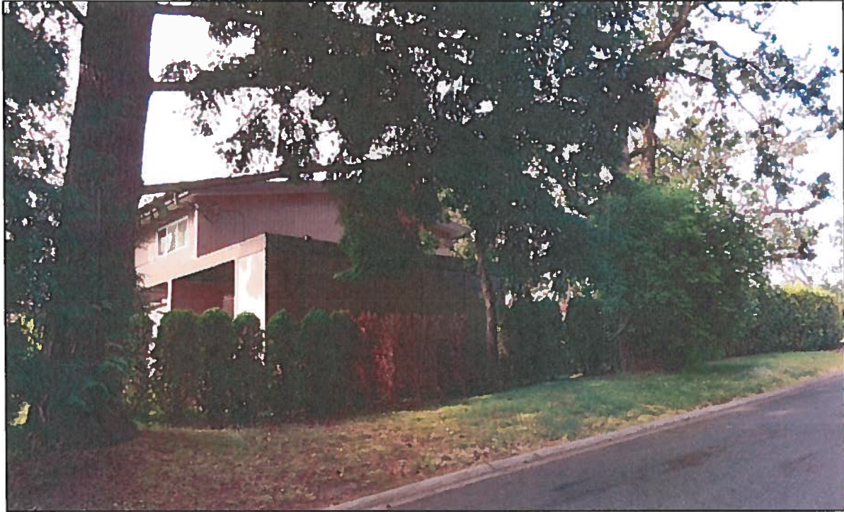
Photograph 3: Looking south at existing carport and dwelling
