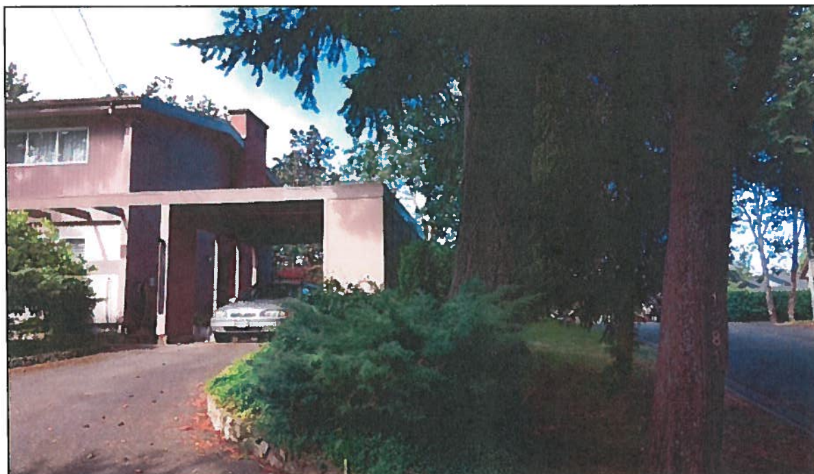
Photograph 2: Looking west from driveway entrance
