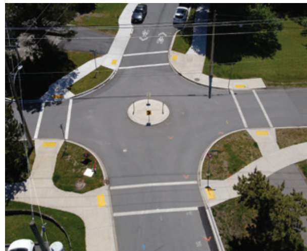
Completed Seaton-Regina sidewalk project
