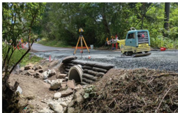
Preparing to pave Charlton Road
