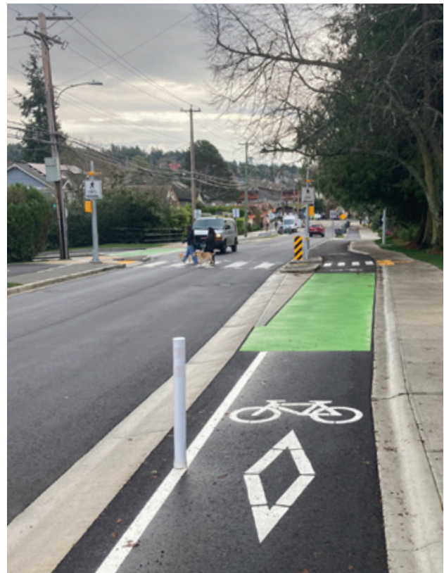
Newly completed crosswalks, sidewalks, and bike lanes on Sinclair
