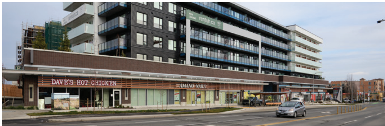
New mixed commercial and residential space near the McKenzie and Shelbourne intersection
