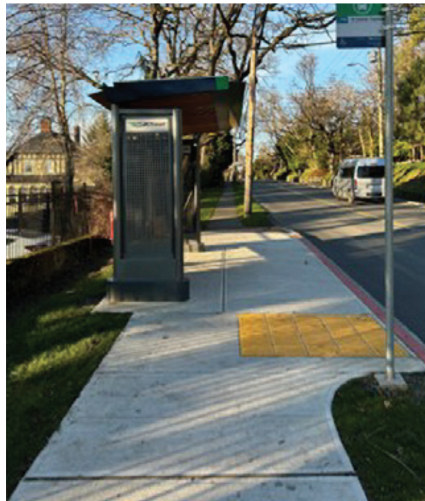
Bus stop improvements at Richmond SB McRae
