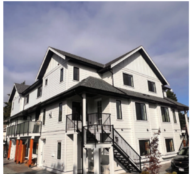
A new fourplex on Epsom Drive provides Small-scale Multi-unit Housing (SSMUH)
