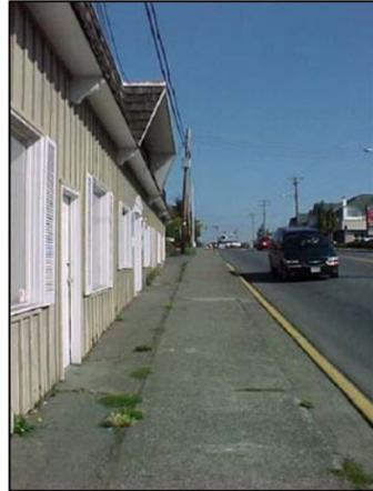
2. Existing sidewalk between Arnot and Vincent Avenue in need of upgrade. Note uneven edge between asphalt patch and concrete sidewalk.
