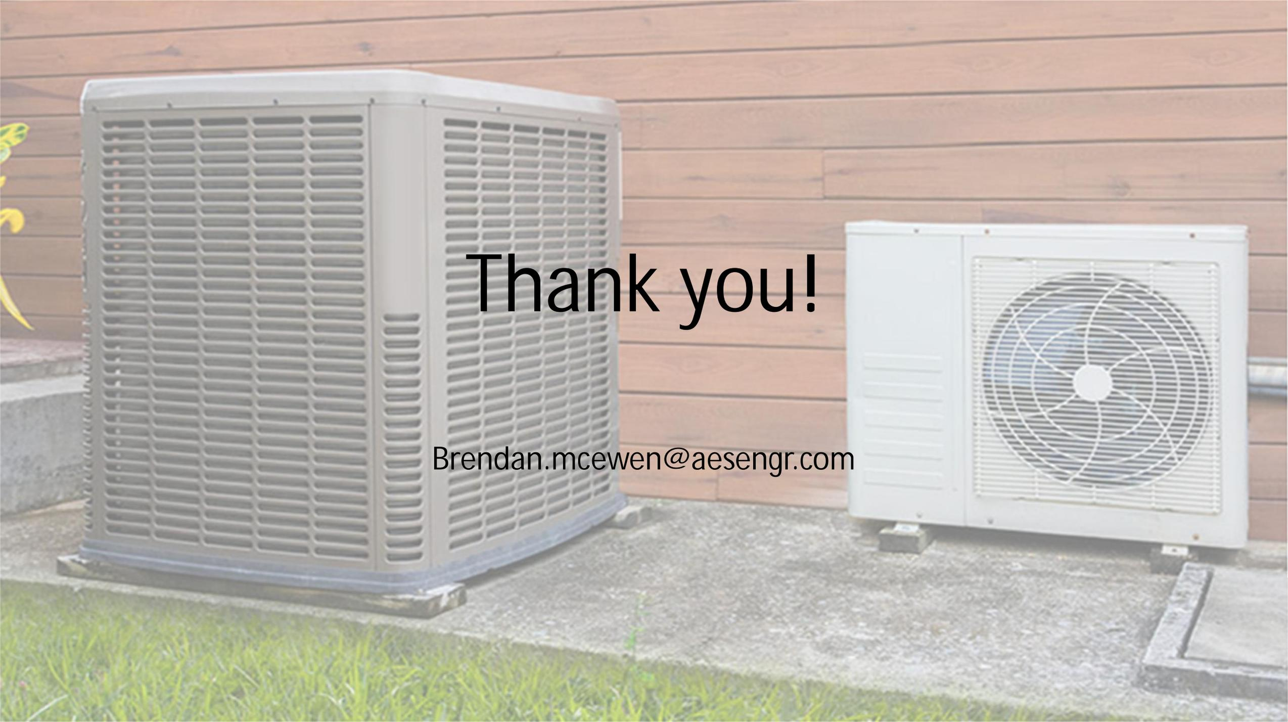
The image shows two outdoor HVAC units against a wood-paneled wall. The unit on the left is a large, grey, rectangular condenser coil unit with a dense grid of slats. The unit on the right is a smaller, white, rectangular outdoor condenser unit with a prominent circular fan grille. The units are mounted on a concrete pad. The background is a wall of horizontal wood siding. The foreground shows a patch of green grass.
