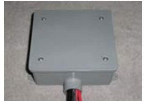
Energized outlet: electric receptacle (6-50R) and outlet box with cover.
