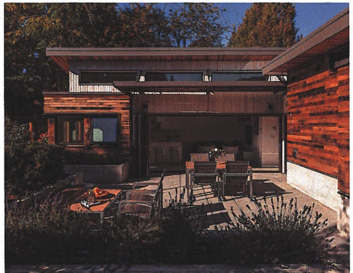
Figure 18: Example of outdoor amenity space with screening for privacy (photo: lanefab.com )
