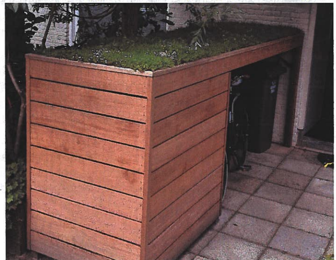
Figure 26: Example of secure and weather protected bicycle parking combined with screened waste and recycling containers
