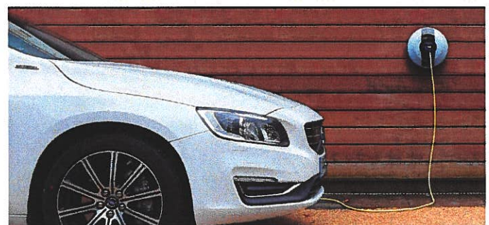
Figure 24: Example of a parking space with an energized outlet for an electric vehicle
