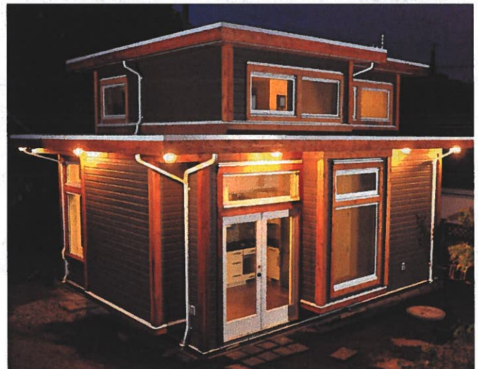
Figure 13: Example of a Garden Suite that is stepped back on the second level to reduce overall massing (photo: smallworks.ca )
