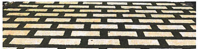
Figure 21: Example of permeable interlocking pavers (Photo: http://www.gtlandscaping.com )
