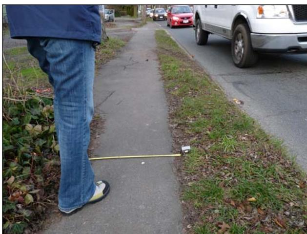
*"Sidewalk" on Shelbourne near North Dairy measures less than one metre in width.*
