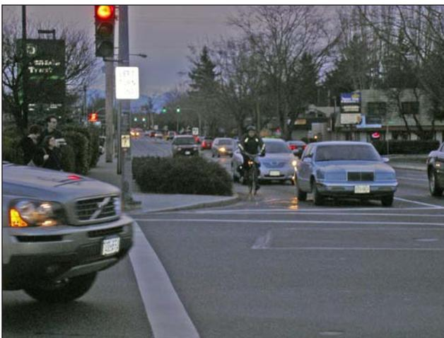
Intersections at Shelbourne and Cedar Hill X Road are dangerous for pedestrians because of heavy traffic and rounded corners, which encourage motorists to turn without stopping.
