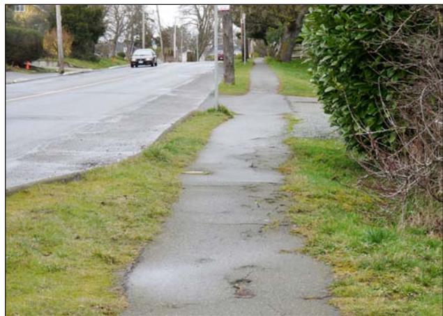
*Deteriorated, broken asphalt sidewalk is typical of that on most of the east side of Cedar Hill Road.*
