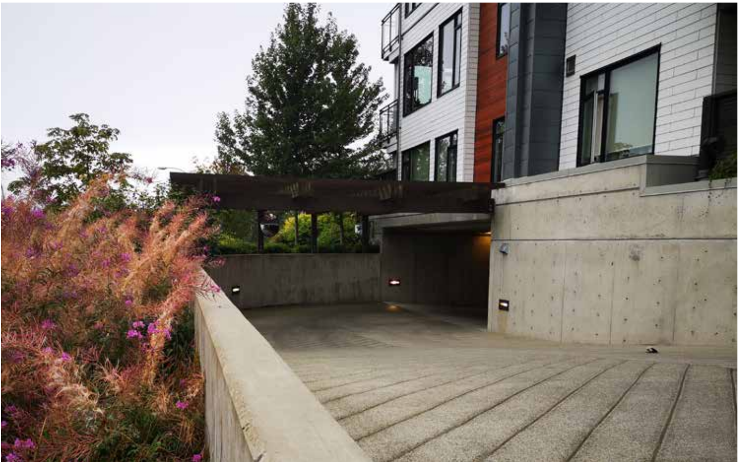
Underground parking off Huxley Street
