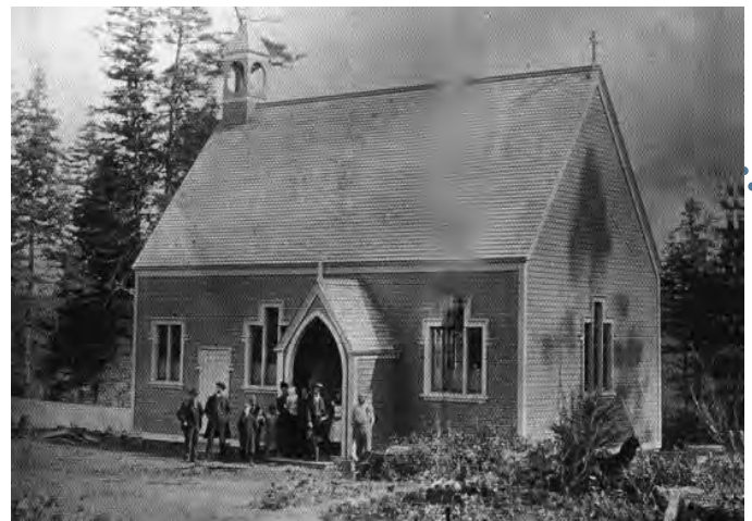
St. Marks Church, 1893.
