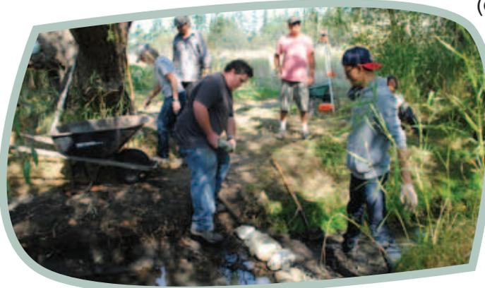
On the Swan Creek site, the channel was previously moved by the Ministry of Transportation and Highways and is devoid of substrate and has very limited riparian vegetation. In December of 2011, a fuel spill in Swan Creek necessitated the construction of a siphon dam in this location. The rock supporting the siphon dam was deliberately chosen as cobble and was released into the channel when the siphon dam was decommissioned in January 2012. Although this riffle
