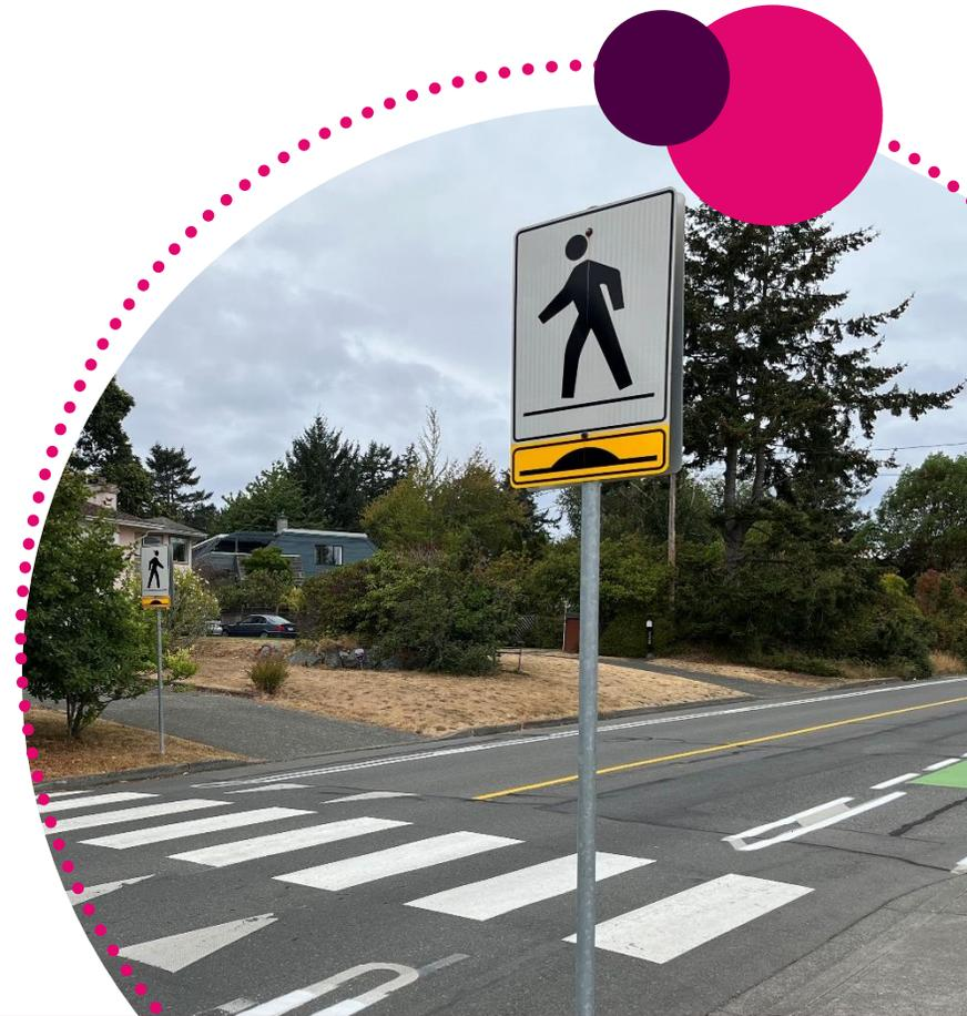
**Raised crosswalks** not only reduce vehicle speeds, but also provide accessibility benefits by allowing crossing to occur at sidewalk level.
