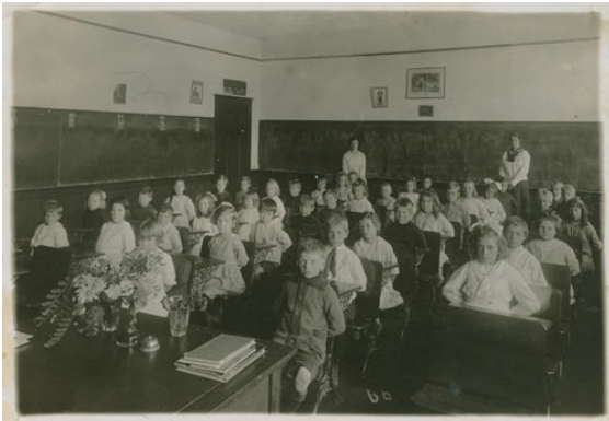
McKenzie Ave. School classroom (2008-016-006)
