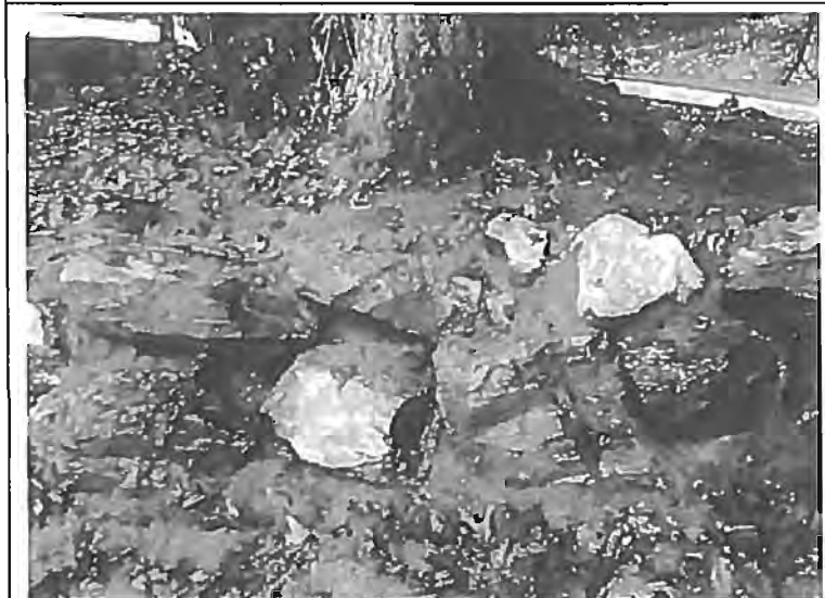
Douglas-fir 710 - Loose stached boulders used to retain upper portion of distribution field. Hand excavation did not encounter any evidence of root damage.
