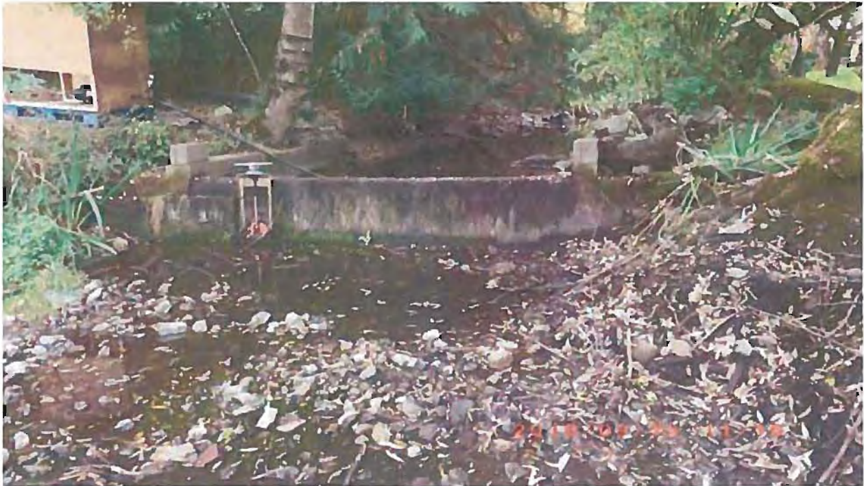
Figure 13. Concrete weir structure downstream of Prospect Lake. This weir was originally installed to provide a seasonal water supply to Butchart Gardens, located downstream on Tod Creek. This weir structure results in Prospect Lake being managed as a reservoir, permitting winter lake volumes to be stored for subsequent release into Tod Creek, during dry summer periods and ensuring that the summer lake level fluctuations are minimized. The weir elevation is 47.03m. The historic high water level is 48.7m, which is 1.67m above the top of the weir.
