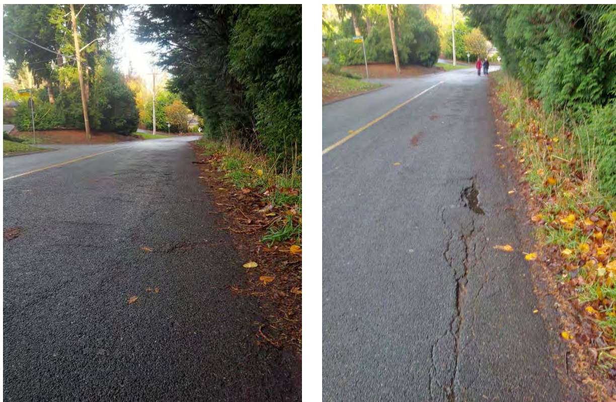
Figure 3: Road surface damage on Del Monte Avenue caused by Leyland Cypress roots
