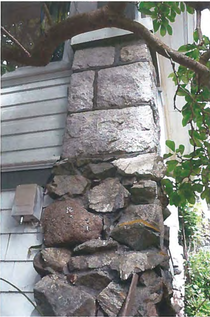
Rubble foundation pillars and granite pillars on porch above
