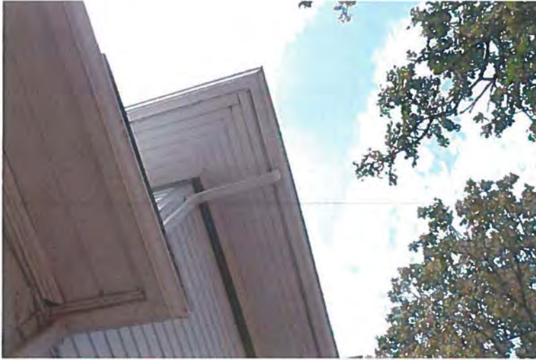
Tongue and groove soffits in eaves
