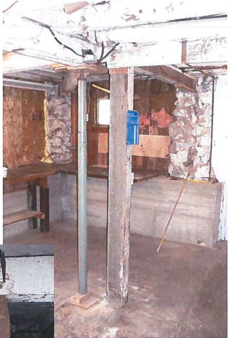
Floor beams, original post support, newer teleposts, rubble foundation pillars, newer concrete addition to extending basement
