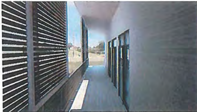
Example of passageway with louvred screen enclosure
