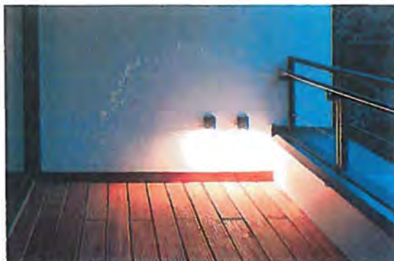
Example of low intensity Exterior Passageway lighting
