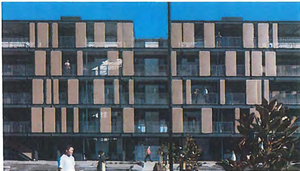
Example of louvred screens on building façade with exterior passageways
