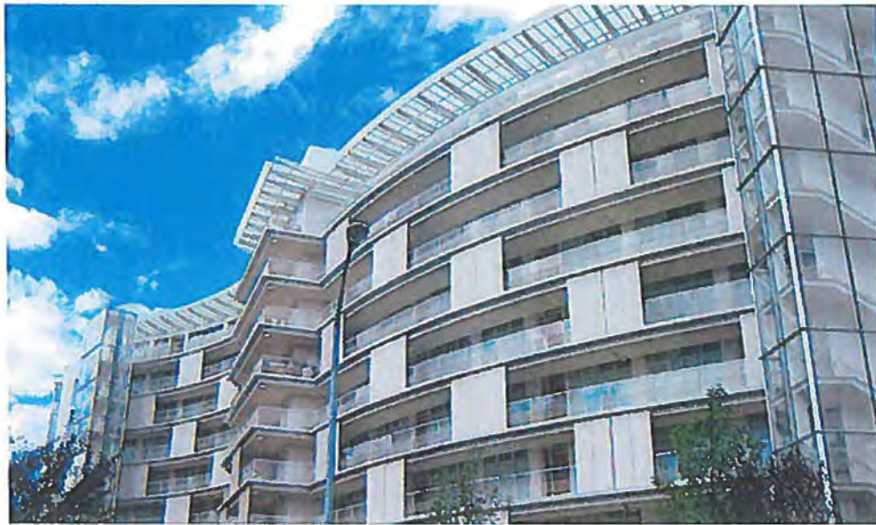
Example of louvred screens on building façade with exterior passageways
