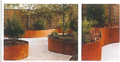
CORTEN RETAINING WALL
