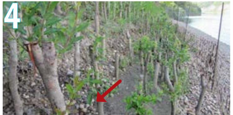
**Photograph 3 and 4.** Dense live staking can be used where erosion is causing a problem. The dense pattern of the live stakes slows the flow velocity of the river and allows sediment to be deposited (red arrow).
