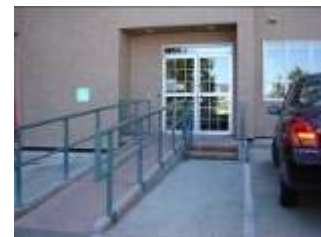
This ramp directs the user into the active parking lot
