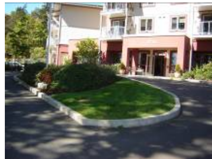
Islands and traffic circles must be designed with the turning radius of handyDART vehicles. Mountable curbs can be used to overcome space restrictions
