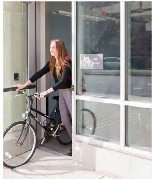
Figure 41: Bicycle room with dedicated entrance (3.4.4. a).
