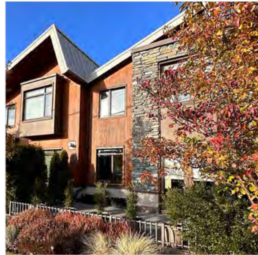
Figure 24: Incorporate substantial, natural building materials such as masonry, stone, and wood into building facades (3.1.6. f).
