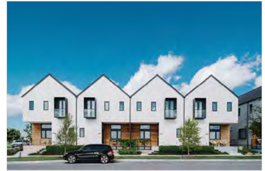
Figure 65: Scale and site buildings to establish by articulating individual units through integration of recessed entries, balconies, a change in materials and slight projection/recess in the facade. (5.1.3. a)
