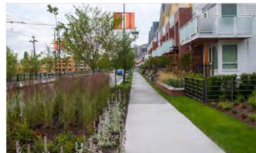
Figure 20: Design sites and landscapes to improve stormwater function by using strategies such as rain gardens and permeable surfacing (3.1.5 p).
