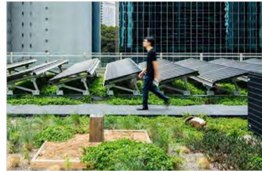
Figure 32: Example of a rooftop with solar photovoltaic array as well as green roof and open space (3.3.1. i).
