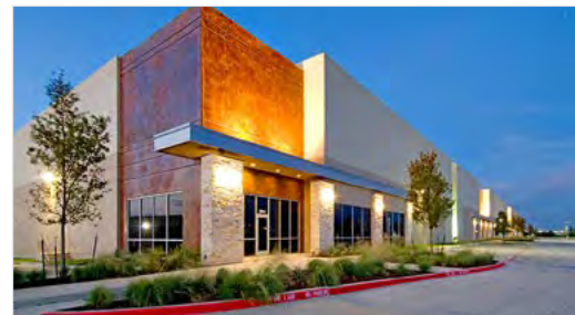
Figure 107: Use of different exterior materials to distinguish between the plant/warehouse component of a building from the office/sales component (9.1.5. b).
