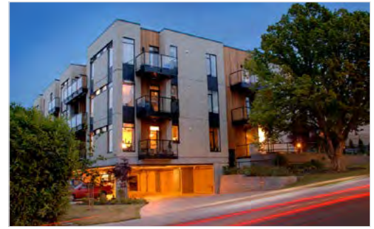
Figure 13: Under building or half underground parking using the slope of the site (3.1.4. j).
