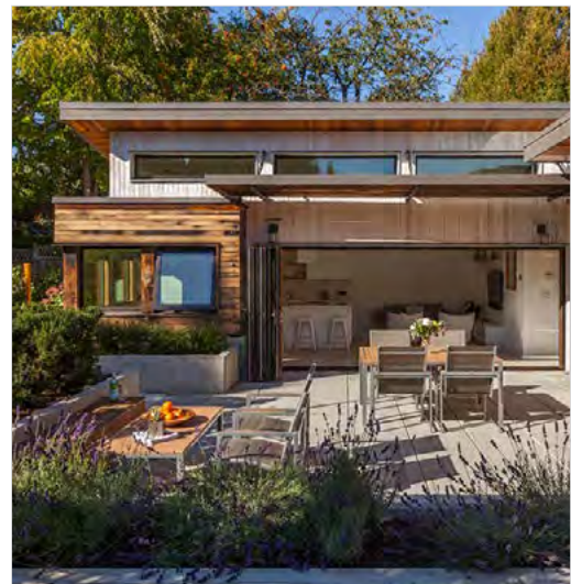
Figure 154: Outdoor amenity space with screening for privacy.
