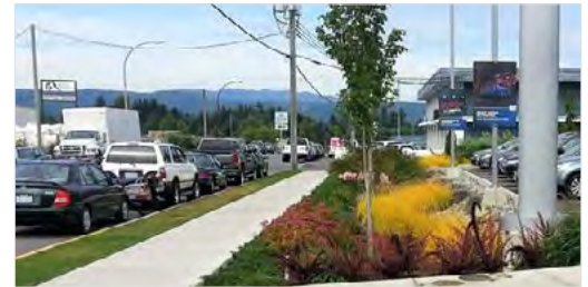
Figure 105: Landscape strip with rain garden adjacent to front visitor parking to provide stormwater management and soften the property edge (9.1.4. a).
