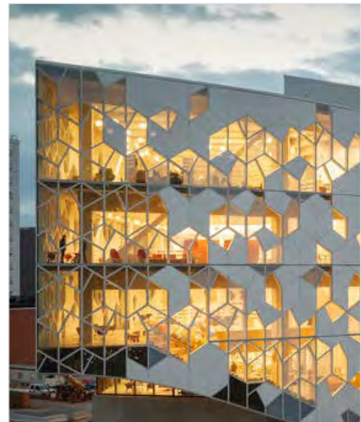
Figure 43: Avoid large areas of glazing where birds can see through them to the sky or habitat on the other side (3.5.1. b).
