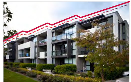
Figure 83: A residential building's roof form is stepped to break up the overall form (6.1.6. f).
