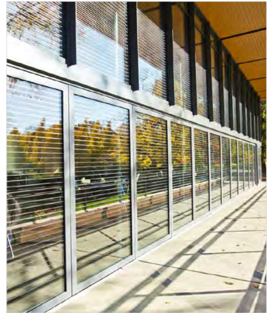
Figure 44: Apply visual markers such as etched glass, ceramic frit, sandblasted glass, and textured glass (3.5.1 d).
