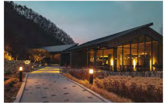
Figure 22: Use full cut-off exterior lighting to complement building and landscape design (3.1.5. s).
