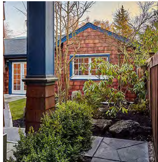
Figure 137: Clear access pathway to a garden suite in the rear yard.
