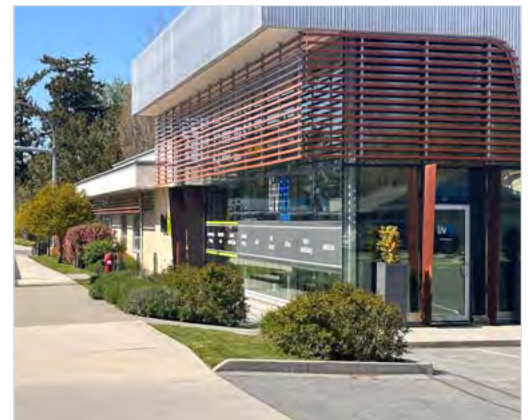
Figure 102: Transparent frontage and use of materiality to indicate units and entries (8.1.5. b).
