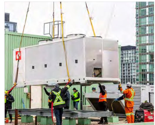
Figure 31: A rooftop heat pump unit being installed (3.3.1. g,h).
