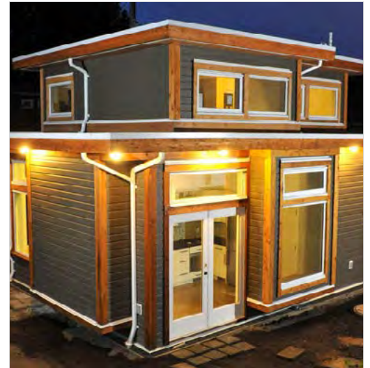
Figure 150: The second storey of a garden suite with a flat or shallow roof steps back and away from adjacent neighbours.
