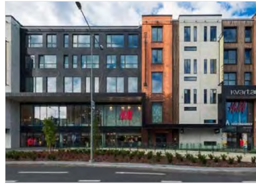
Figure 77: Buildings over 40 m in length should incorporate a significant horizontal and vertical break in the facade (6.1.3 a).
