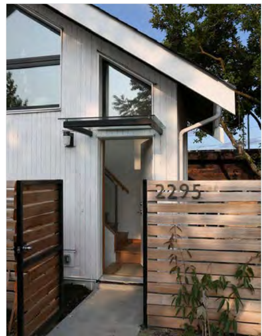
Figure 148: A covered entry to a garden suite provides weather protection.
