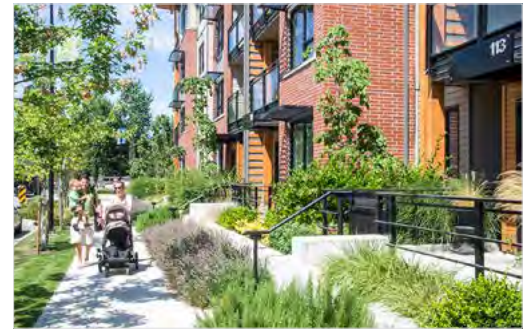
Figure 78: Example of a raised residential frontage with semi private patios over half underground parking (6.1.4. c).
