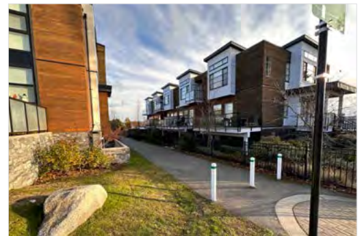
Figure 63: Townhouse projects that have internal circulation and connectivity should have building entries that face onto the paths in order to create an active edge (5.1.1. b)
