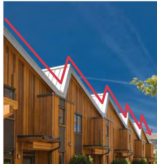
Figure 72: Use of roofline features as a strategy for articulating individual units (5.1.6. a).
