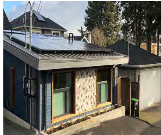
Figure 153: Potential to support solar panels.
