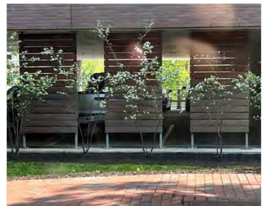
Figure 16: When provided at grade, screen or enclose parking to minimize view and impact on the public realm (3.1.4. m).
