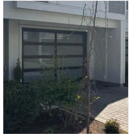
Figure 53: Minimize impact of garage doors by recessing them into the facade (4.1.4 e).
