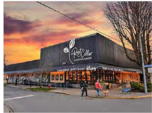
Figure 100: Buildings on a corner parcel should orient frontages towards both streets if possible (8.1.2. a).
