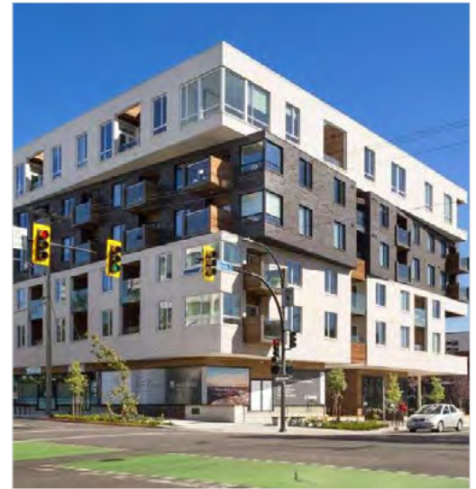
Figure 82: Articulate the facade using design elements that are inherent to the building as opposed to being decorative (6.1.6 e & f).
