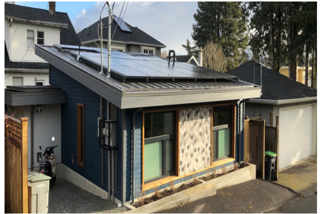
Figure 18: Potential to support solar panels
