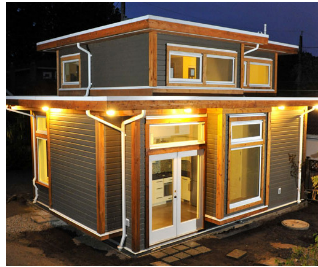
Figure 15: The second storey of a garden suite with a flat or shallow roof steps back and away from adjacent neighbours
