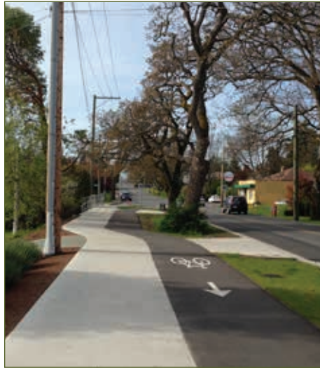
Existing Cycle Track on Cedar Hill Road
