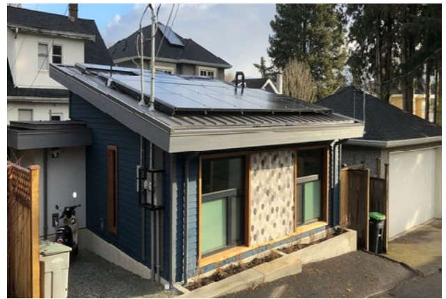
Figure 18: Potential to support solar panels
