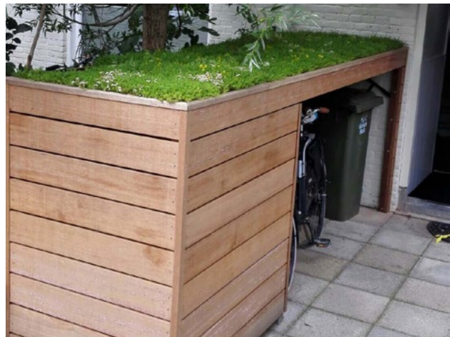
Figure 27: Screened waste and compost containers
