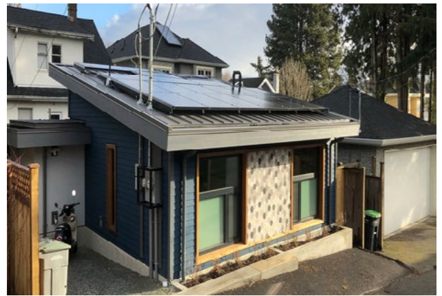
Figure 18: Potential to support solar panels
