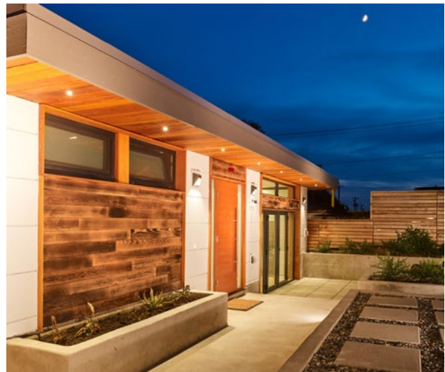
Figure 11: Fully-cut off light fixtures create a safe environment with minimal light spill
