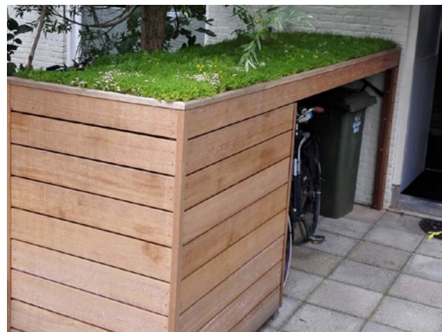
Figure 27: Screened waste and compost containers
